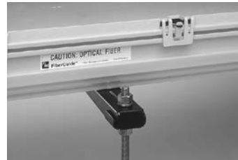
Straight Section Cover Attached to Straight Section
